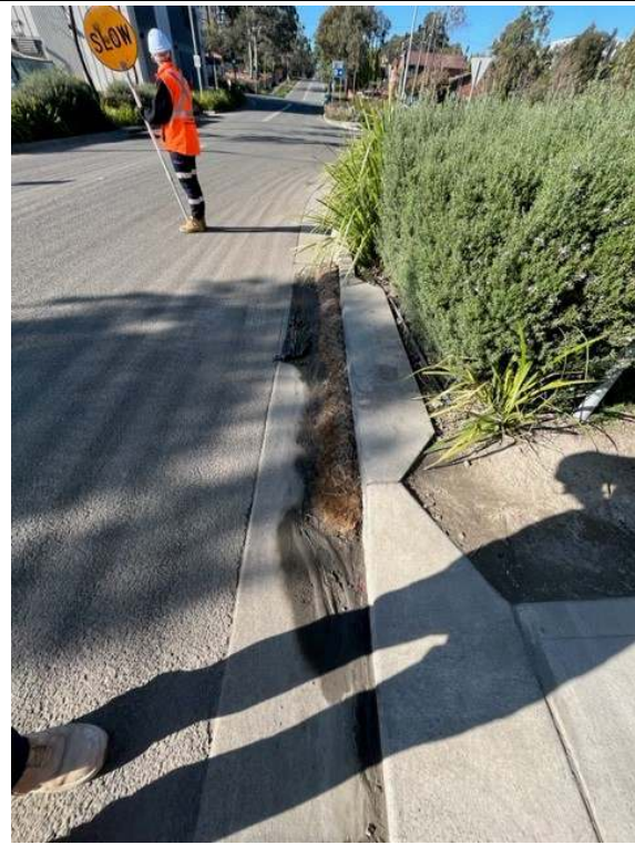
Photos 19 & 20: Concrete pour and ERSED controls requiring replacement on Andalusian Way
