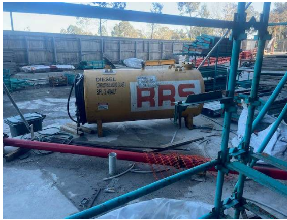
Photo 15: Diesel storage tank for cranes – spill kit required
