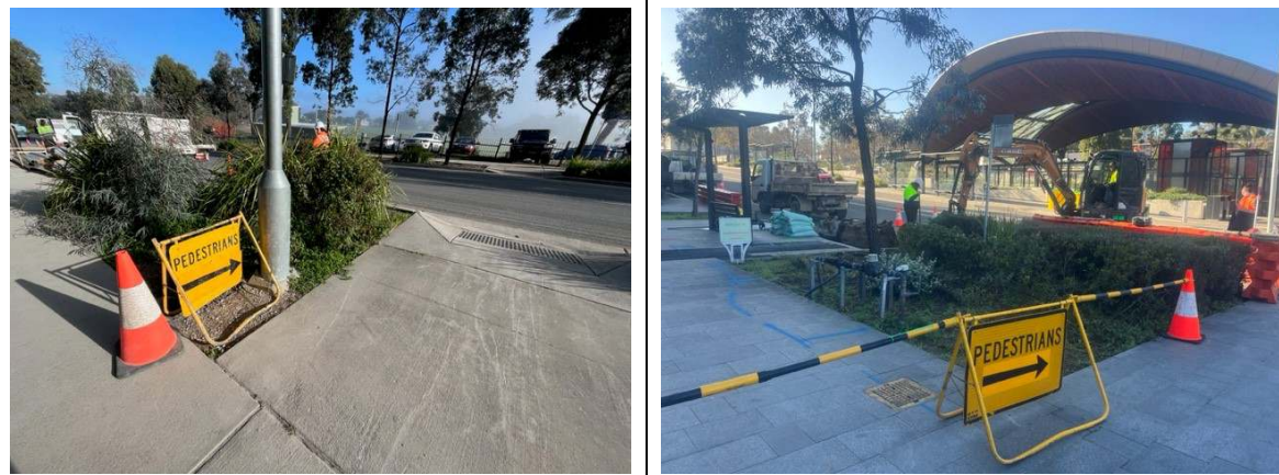
Photos 3-6: Traffic control and pedestrian diversion signage setup around the site
