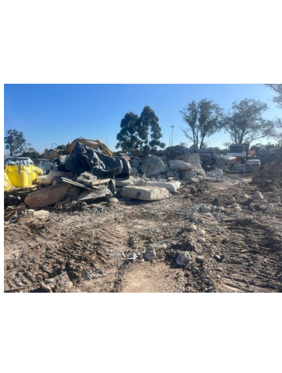
Photos 23-26: Build-up of bulldust across the site compound hardstand presenting potential dust risk. Stockpiling and waste storage for recycling / disposal offsite by Aussie Skips.
