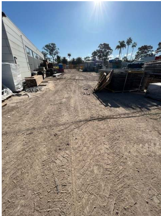
Photos 23-26: Build-up of bulldust across the site compound hardstand presenting potential dust risk. Stockpiling and waste storage for recycling / disposal offsite by Aussie Skips.
